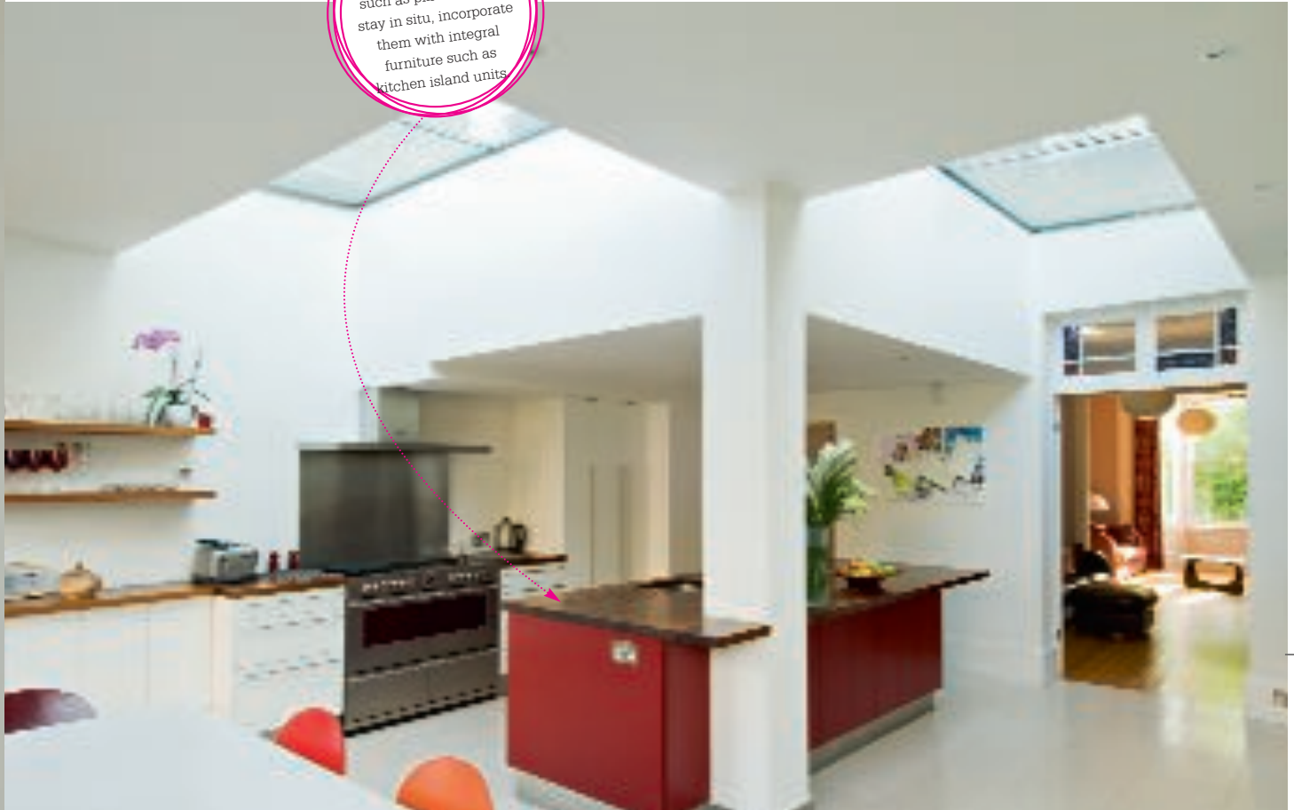
Above: There was little room for error when it came to installing edge glass to edge glass in the frameless rooflights. Glass can't be planed to fit, it must be spot on.
